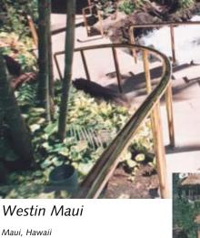
Architect: Lawton Umemura Architects Bright Finish Brass 2" O.D. One-Line Floor Mounted Rail (51mm) Model # U-200-1/BB
